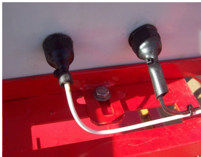
Figure 18 Sealing of antenna and power supply inputs.
