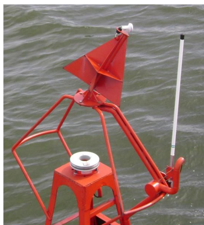
Figure 7 Antenna damage due to collision
