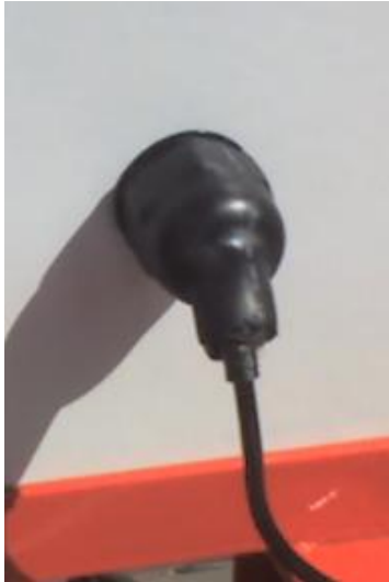
Figure 19 Sealed cable gland with heat shrink
